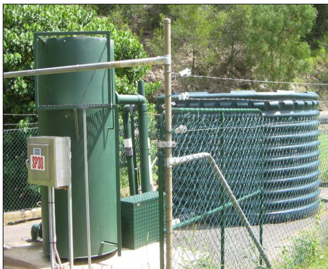
Plate 2.1 Scaled up demonstration pilot plant at Hinze Dam showing the fluidisation column and tank for recycle batch tests. Source: Okamura, et al. (1996).
